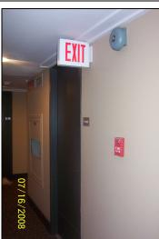
View of the typical illuminated exit sign, alarm bell, pull station, and fire hose cabinet adjacent to the exit staircase in the common area hallways at the Subject Property tower building. Above the hose cabinet is a fire strobe light and ionization detector.
