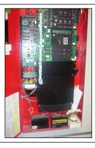
Close-up view of the fire panel located in a small room adjacent to the common area lobby at the tower building; note the battery backup cells at the bottom of the panel.
