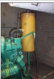
View of the water cooling tank at the diesel-fired emergency generator, located in level #B-1.
