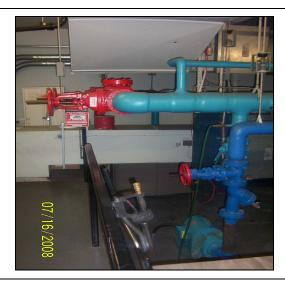
Another view of the shut-off valves at the high pressure domestic water supply line (light blue) located in the basement mechanical room. Management indicates that the valves are original, not totally effective and should be replaced.
