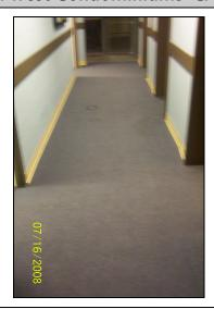
View of the common area hallway servicing the laundry room and elevator lobby at level #B at the tower building at the Subject Property; note the carpet is showing signs of wear and is stained at this high-traffic hallway.
