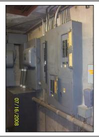
Close-up view of the sub panels located in the electrical room, level #B-1; sub panels shown are connected to level #B equipment including receptacles, lights, trash compactor and landscaping controls.
