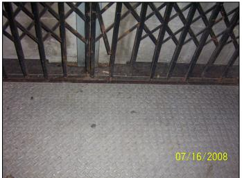
View of the freight elevator accordion door and diamond plate floor sheeting; the door is bent from impact, is difficult to operate and needs repair or replacement.
