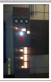
View of the automatic controls monitoring the water discharge, and suction pressures, with shut-off switches for all three of the water pumps, located in the mechanical room, floor #1 of the tower building.
