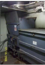
View of the refuse compactor located in a closet at the tower building; note the trash chute termination above the hopper; there is no disinfectant system installed within the chute.
