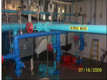
View of the fire pump (red) the low pressure domestic water supply line (dark blue) and the high pressure domestic water supply line (light blue) located in the basement mechanical room, floor #1, in the tower building. All three sets of the shutoff valves on the domestic and high pressure water lines need replacement, according to management. The automatic sprinkler system valves that shut-off the high pressure lines are newer and in good condition, according to management.
