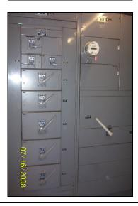
View of the primary power main rated at 1200 amp, and disconnect switches located in the electrical room level #B-1, adjacent to the parking garage in the tower building at the Subject Property; the primary transformer room was locked by the providing utility company.
