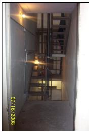
View of the firemen's staircase to the roof; stair stringers and handrails are painted metal and treads are expanded metal mesh, while landings are unpainted concrete.
