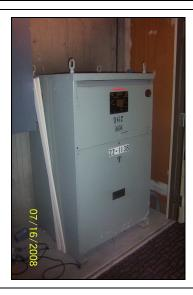
View of a typical electrical step-down transformer, this one located in a typical common area hallway closet; transformers occur in these closets every third floor.
