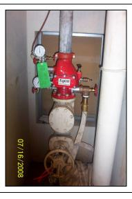
View of the inspection tag, gauges and valves on the dry fire sprinkler riser system installed in the garage, level #B-3.
