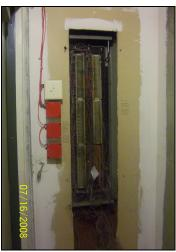
View of the typical telephone communications panels located in closets adjacent to the common area hallways at every third floor, at the Subject Property tower building. The red cover plates are junction boxes for fire alarm hardware. The long vertical box houses active telecommunications wiring.
