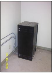
View of the amplifier for the fire alarm system speakers and enunciators located in the fire panel room adjacent to the lobby in the tower.
