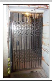
View of the freight elevator accordion door; the door is bent from impact and needs repair or replacement.
