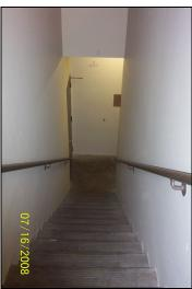
View of the typical common area exit door staircase at the Subject Property tower building; stairs are bare, unpainted concrete and walls and ceilings are painted concrete, plaster or wallboard.
