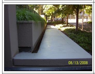
Close-up view along SW Third Avenue, looking south, of the gutter at the retaining wall below the planter shown in the previous photos; note the presence of standing water.
