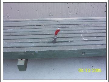
Another view of the wood bench shown in the photo above; the author's knife blade was also easily inserted into the 2x4s at this location indicating the presence of rot.
