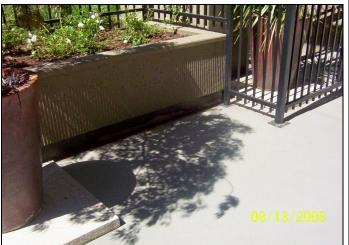
View of the east side of the west planter at the west plaza, adjacent to the west entry gate, looking northwest; note the dark membrane above the gutter is peeling.
