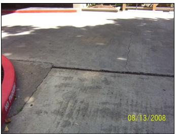
Another view of settled concrete and fractures in the slabs at the east side of the porte cochere at the main entrance into the tower, building #1; displaced slabs represent a tripping hazard.
