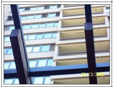
Close-up view of the trellis wood components at the west entrance gate; note the lack of sheet metal caps at the ends and tops of the wood cross struts.
