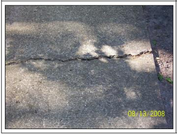
View of the cracked driveway into the parking garage.
