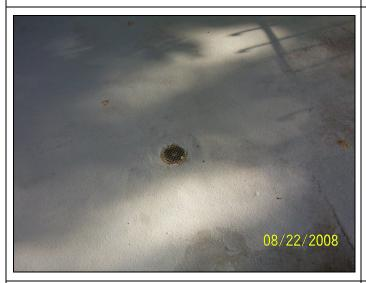
View of the typical area drain in the plaza with the liquid waterproof membrane coating where it appears some drains have been added in areas of concrete creep.
