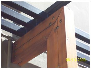
Another view of the trellis at the west side of the main entrance into the tower building #1; the beam and post appear to be checking. The lack of sheet metal caps at beam tops and the possibility that water penetration may occur at all such cracks and at the mitre joint between beam and post may result in advanced deterioration of the assembly.
