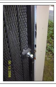
View of the steel jamb at the northwest exit gate shown in the previous photo; the gate is rubbing on the jamb exposing bare metal.
