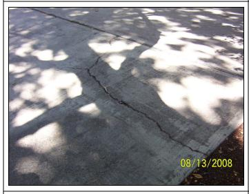
View of cracks in the curb-cut apron into the porte cochere driveway at SW Harrison Street, at the east side.
