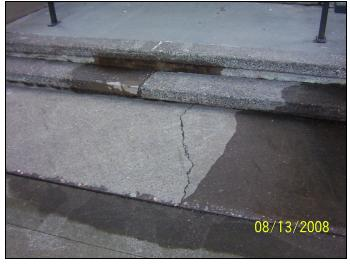
Close-up view of the crack in the lower landing of the stairs shown in the previous photo.
