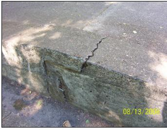
View of cracked concrete retaining wall sections of the ramp into the parking garage, this on the west side.
