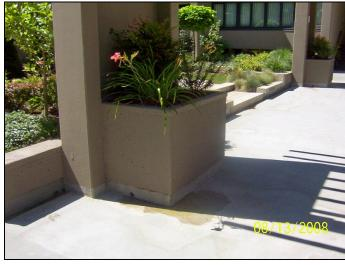
View of the stains on the waterproof surface from the opposite planter box in the previous photo; note the open gutter around the raised planter.
