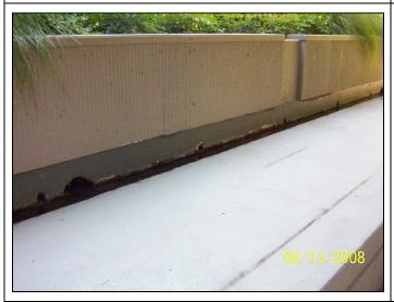
Close-up view of the gutter at the base of the planter retaining wall shown in the previous photo; note the peeling coating above the gutter.
