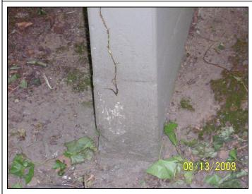
View of a concrete stem wall at the north façade of building #2, between units #2 & #3; note the coating is peeling.
