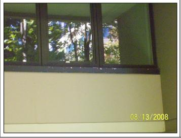
Close-up view of the coating peeling on sheet metal flashing below window frames shown in the previous photo, building #2, unit #1.
