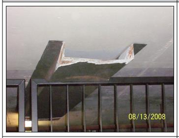
View of an exhaust duct surface applied to the parking garage soffit below unit #3, building #2; note the corrosion on the end
