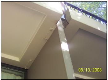
View of the north end of the soffit at building #5, unit #12; the steel shelf angles appear to be rusting.
