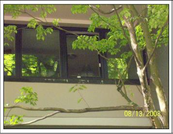
View of the coating peeling on sheet metal flashing below window frames at the west end of unit #6, building #3.
