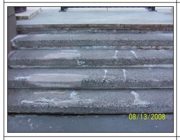
Close-up view of the concrete stairs at the plaza west entrance from SW Third Avenue; note the extensive patchwork on the tread surfaces and nosings. Also, the steel angle at the top tread nosing is rusted.
