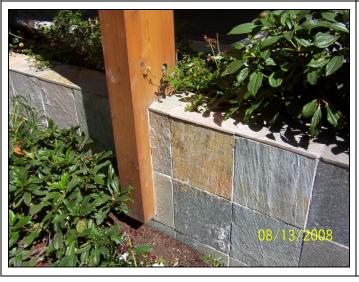
Close-up view of the planter and trellis at the south side of the main entrance into the tower, building #1; the wood post appears to be making contact with the planter tile which may result in premature degradation of the wood.
