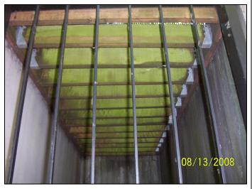
View of the 2x6 wood joists supporting a steel grate above the northwest exit gate shown in the previous photo; the joists and ledgers are supporting algae growth but appear to be pressure treated.
