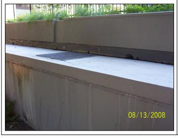
View of the metal fencing, planters and retaining walls along SW Third Avenue, north of the west entrance gate; note water seepage on the retaining wall, under the top slab. The steel grille on the concrete lid appears to be the exhaust from one of approximately four parking garage exhaust fans.
