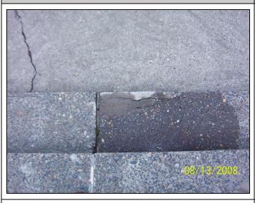
Close-up views of a cracked and patched tread, and crack in the bottom landing of the stairs shown in the previous photo; the tread patch appears to be cracking.
