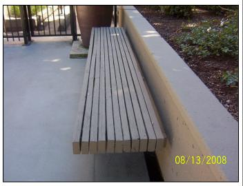
The bench at the sitting area at the south end of the west plaza shown in the previous photo did not appear to have rot in the 2x4s, but 2x4s are warped and prevent debris from falling through that can promote rot.
