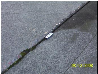
View of ½" settlement between the concrete slab landing and the public sidewalk shown in the previous photos, representative of tripping hazards; this slab has received prior grinding and needs to be done again.
