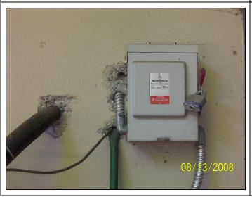
View of the Westinghouse disconnect switch servicing the condenser providing air-conditioning to the maintenance shop; note the wall penetrations have been not been sealed or grouted shut.
