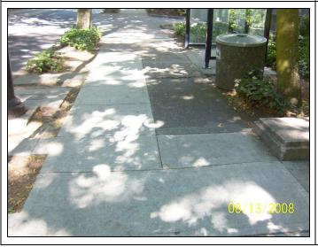
The public sidewalk along SW Harrison Street, in front of the Tri-Met Enclosure, has buckled and received various repairs.
