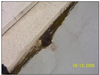
View of a control- or seismic-joint at the east plaza; there appears to be a rubber membrane with flat metal bar between slabs, both sides of the area drain.
