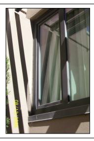
Close-up view of the typical unit window; windows are fixed or are combination awning/sliding (at first floor living rooms only, casement elsewhere) frame types. Frames appear to have been inserted into the rough openings and caulked all around, with a sheet metal flashing installed at the head and sill.
