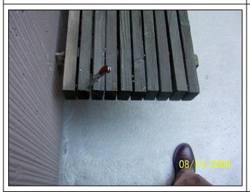
View of the wood bench at the sitting area adjacent to the exit staircase from the north plaza between buildings #1 & #2; note the author's knife blade easily inserted into the 2x4s indicating the presence of rot.
