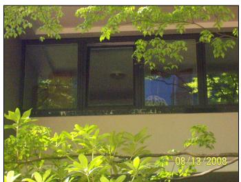
View of the coating peeling on sheet metal flashing below window frames at the east end of unit #6, building #3.
