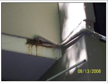
View of corrosion above the soffit at a pipe penetration, above the light fixture shown in the previous photo.
