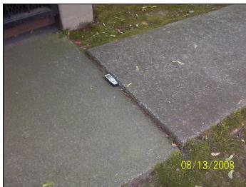
View of settlement between the concrete slab landing and the sidewalk to the northwest exit gate shown in the previous photo; note the author's digital recorder indicating an approximately 1" settlement between slabs, representative of a tripping hazard.
