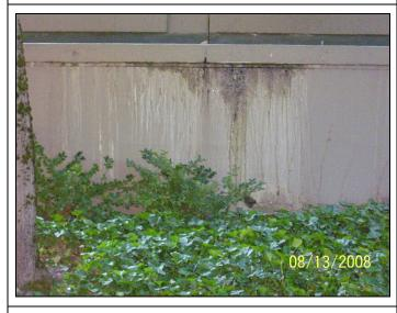
Close-up view of water and efflorescent stains on the retaining wall below the planter shown in the previous photo.
