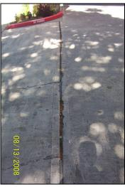
View of the crown into the porte cochere driveway at SW Harrison Street, at the east side. The apron is cracked and the slabs have settled differentially, creating tripping hazards.
