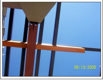
View of the wood trellis connection to the concrete wall, typical at the plaza; note the lack of sheet metal caps on the top of the wood components.
