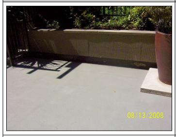
View of the east side of the west planter at the west plaza adjacent to the tower building #1, looking west; note the dark membrane above the gutter is peeling.
