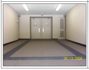
View of the exterior covered entry at the east side of the tower building #1; note the CCTV security camera above the door head. Outdoor carpeting appears to be in good condition. The staircase on the left accesses levels #B-2-#1, while the right side accesses levels #1-#26, with access to the roof.
