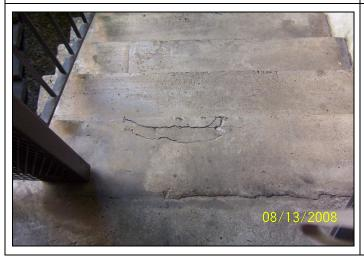
View of a damaged tread surface that has been patched but is again cracked on the first tread from the top parking garage level to the bottom parking garage level at the northeast staircase.
