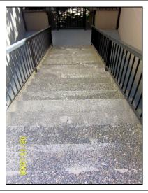
View of the exit staircase from the plaza between buildings #4 & #5, looking east; note the numerous patches and repairs to the treads and nosings.
