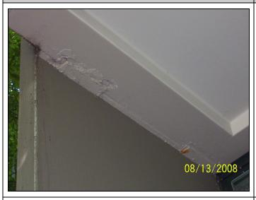
View of the south end of the soffit at building #5, unit #12; the steel shelf angles appear to be rusting slightly beneath the
