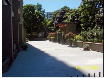
View of the north end of the north planter at the west plaza adjacent to the tower building #1, looking southwest; note the dark membrane above the gutter is peeling.
