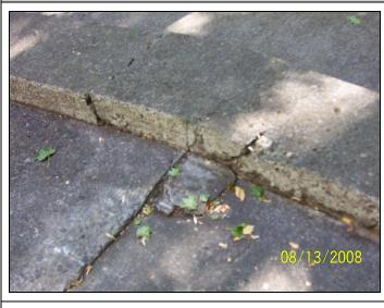
View of cracked concrete driveway and retaining wall sections of the ramp into the parking garage, this on the east side.
