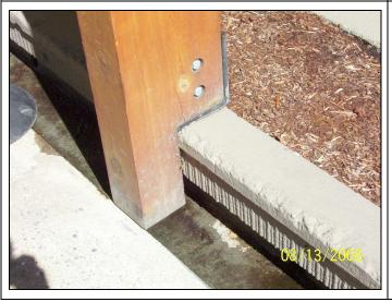
Close-up view of the trellis at the east side of the main entrance into the tower building #1; the wood appears to be held up off the concrete planter, driveway and gutter.
