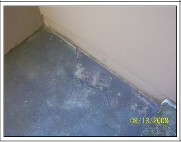
View of the northeast exit staircase from the east plaza, looking at the first landing; note the coating appears to be peeling and delaminating.
