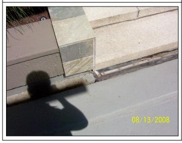
Another view of a control- or seismic-joint at the east plaza; note the flat metal bar on the rubber membrane between slabs.
