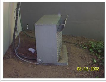
View of the condenser that provides cooling to the maintenance shop shown in the previous photo; note the unit appears to be out of plumb on the sheet metal curb.
