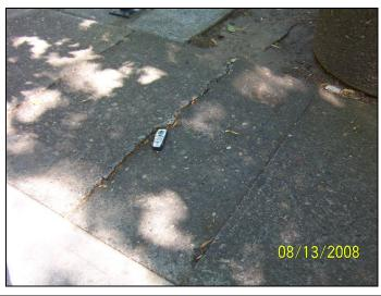
View of cracked and displaced sidewalk panels that represent tripping hazards that should be repaired or replaced; the author's digital recorder is approximately 1" thick.
