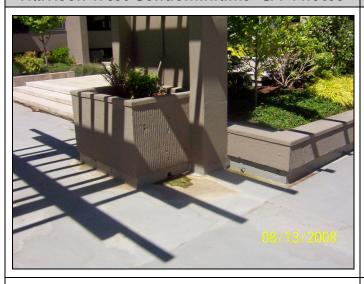
View of the stains on the waterproof surface from the planter box; note the open gutter around the raised planter.
