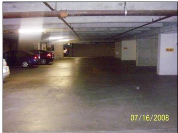
Another view of the parking garage in the tower building; note the fire sprinkler system, a dry system charged with compressed air.
