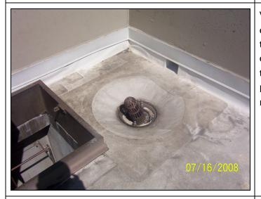
View of the roof drain in the northwest corner of the elevator penthouse roof; note the strainer cap is tilted and should be corrected. Also note the parapet scupper to the right of the drain and the several patches on the single ply roofing membrane.
