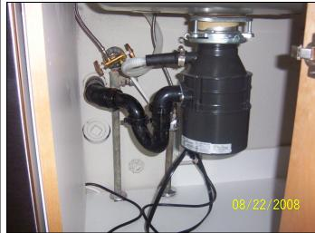
View of the typical under-counter kitchen plumbing in the townhouse buildings; note the unpainted galvanized water supply piping.
