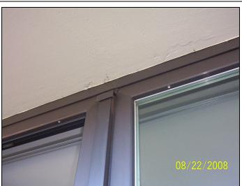
View of the head and jamb of the typical metal window frame at the movable section, typical at floors #2 through #26, at the tower building; the head is covered by a metal flashing and appears to be caulked at the top edge. The movable section functions as an awning window or as a casement door, operable by a single handle.
