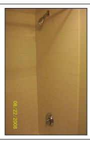
View of the bathroom tub/shower enclosure plumbing; supply lines from the wall to the fixtures are chromium plated metal.
