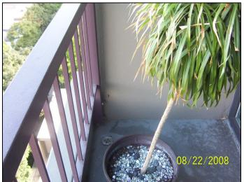
View of another deck floor drain at the opposite end of the deck shown previously; all drains extend to daylight below the soffit of the deck below. The liquid membrane on the deck terminates at the bottom of the concrete end walls and front curb. The metal handrail was re-coated in 2006, according to management; also note the railing is attached to the inside vertical face of the curb and not to the end walls or the deck.
