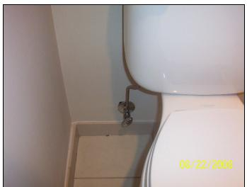
View of the bathroom water closet plumbing; supply lines from the wall to the fixtures are chromium plated metal.
