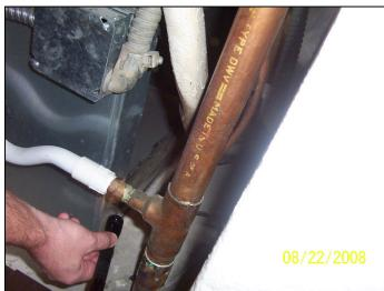
View of the copper condensate drain pipe that runs through the tower building vertically in the furnace closet.
