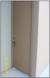
View of the typical townhouse entry door; all unit doors are metal solid core flush panel doors set into steel frames.
