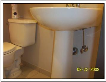
View of the bathroom lavatory plumbing; supply lines from the wall to the fixtures are chromium plated metal.
