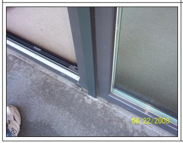
View of the sill and jamb of the typical metal window frame at the movable section, typical at floors #2 through #26, at the tower building; the sill of the frame appears to be raised approximately ½"-1" above the deck, is caulked, and has weep holes for frame drainage. The occupant indicated no leaks have occurred. The movable section functions as an awning window or as a casement door, operable by a single handle.
