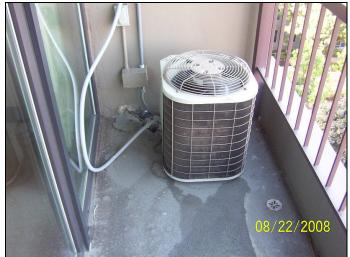
View of the typical air-conditioning condenser installed at each deck; owners were given the option of upgrading their heating system. This appears to be one of the older condensers. Also, note the deck floor drain that appears to be above the drainage pattern on this deck; decks were coated with a liquid waterproof membrane with integral grit in 2006, according to management.
