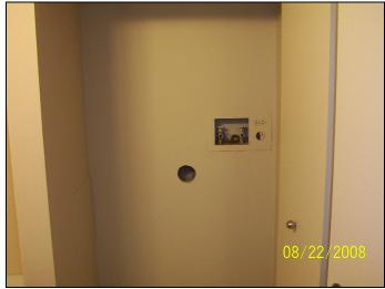
View of another typical laundry manifold installation for supply, waste and power, this one in the townhouse units; note the dryer vent.
