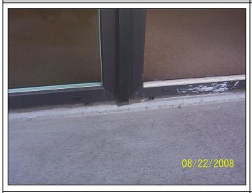
Another view of the sill and jamb of the typical metal window frame at the movable section, typical at floors #2 through #26, at the tower building; the sill of the frame appears to be raised approximately ½"-1" above the deck, is caulked, and has weep holes for frame drainage. The occupant indicated no leaks have occurred. The movable section functions as an awning window or as a casement door, operable by a single handle.
