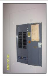
View of the typical electric sub-panel present in each unit; each unit sub-panel is rated at 225 amp, 120/240 volt,  $1\Phi$ , 3-wire, according to management, but disconnect switches at meters indicate that unit service is limited to 150 amp.
