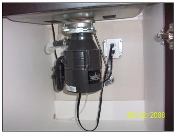
View of the under counter kitchen plumbing in unit #26-B; waste lines are ABS and supply lines are galvanized iron within walls and a combination of stainless steel wire mesh rubber tubing and translucent PEX within cabinets and chromium plated metal where exposed.
