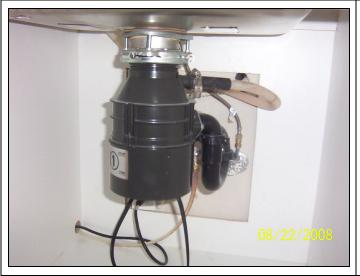
View of the under counter plumbing in unit #10-C; waste lines are ABS and supply lines are galvanized iron within walls and a combination of stainless steel wire mesh rubber tubing and translucent PEX within cabinets and chromium plated metal where exposed.
